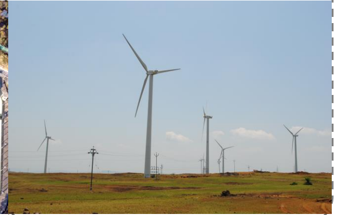
Khirvire Wind Power Station
